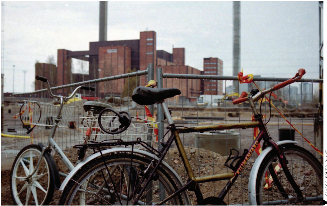
CLASSY POWER PLANT
